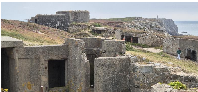
Bunker Pointe de Pen Hir
