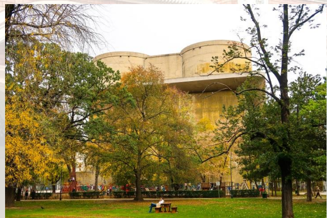
Foto 8 Flak tower VIII - G-Tower Vienna
